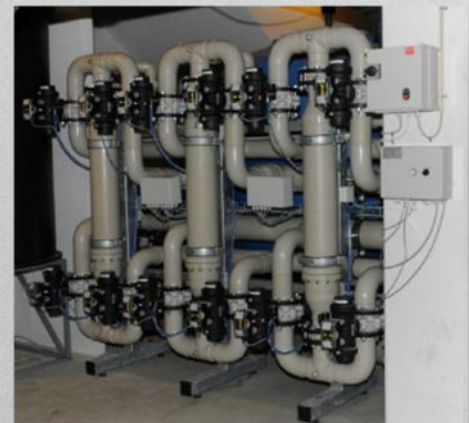
Figure 2: Membrane installation delivered by Provital Solutions
